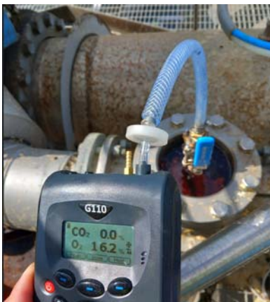
Figure 8. Sampling point and measurement for the residual gas in reactor 2.
